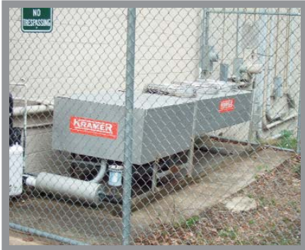
For this installation, the chain link fence surrounding the unit was moved away from it to allow for adequate air flow. Please contact your local HVAC service person to make sure that if you install an enclosure around your machine, it will not have a restricted airflow. Once the fence was installed, final measurements were taken and the panels were fabricated. The installers held the panels to the fence by using exterior grade zip-ties through the grommets that were installed across the top, middle and bottom of the panels during manufacturing.
