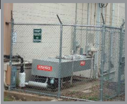
Machinery noise can be an extremely annoying problem. Any noise source that is set onto a concrete slab and backed with concrete block is going to sound many times louder than it actually is due to the reflection of all of the noise in one direction. In order to fix this problem, a line of sight barrier must be constructed and it is strongly advised to introduce some absorption onto the reflective surface of the building "behind" the machine.
